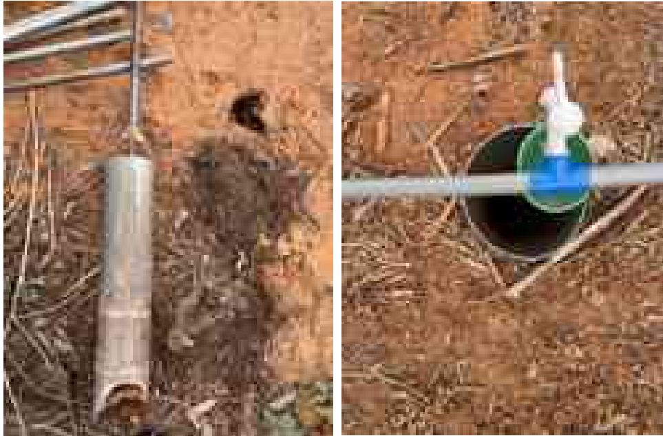
Figure 12-6: Auger and Injection Hole
