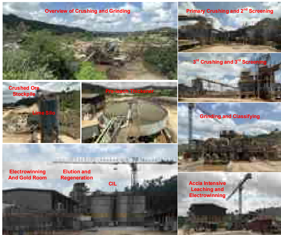
Figure 13-2: Photo of Wassa Processing Plant
