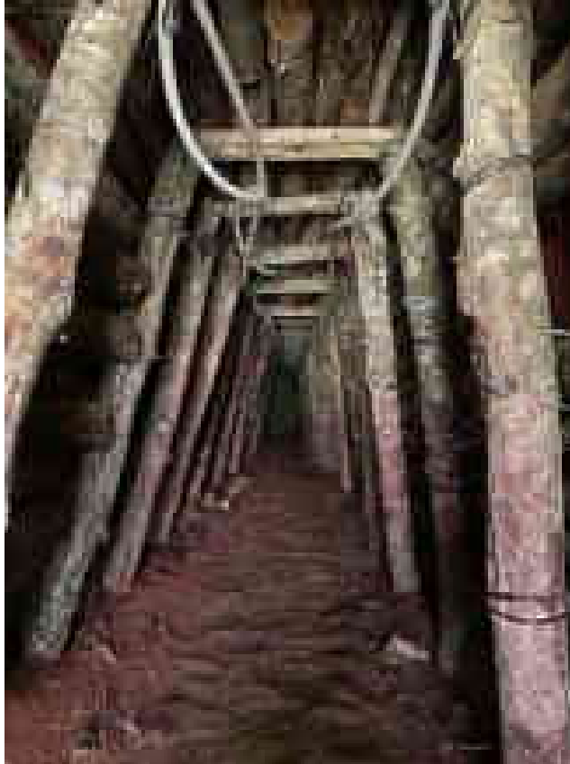
Figure 12-7: Main PLS Collection Tunnel in Construction
