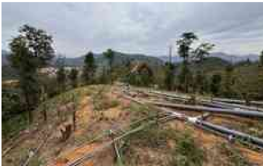
Figure 11-2: In-Situ Injection System at The Mountaintop
