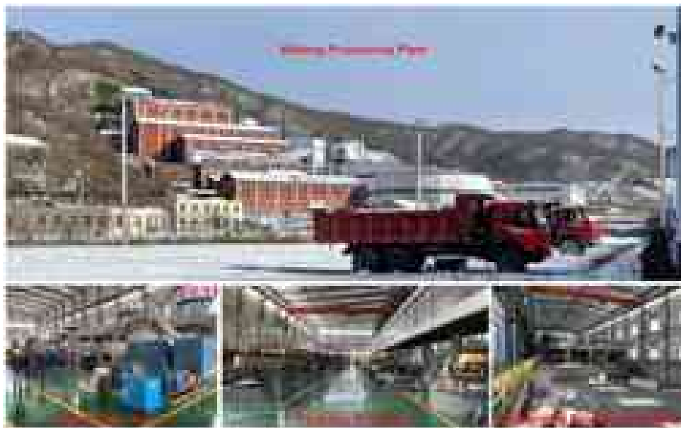
Figure 11-9: Site Photos of Wulong Processing Plant
