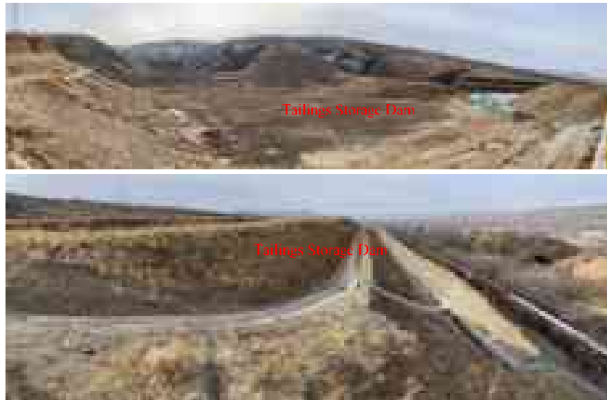
Figure 11-7: TSF of Huatai Mining
