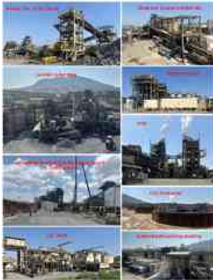
Figure 13-3: Facilities of Sepon Gold Plant
