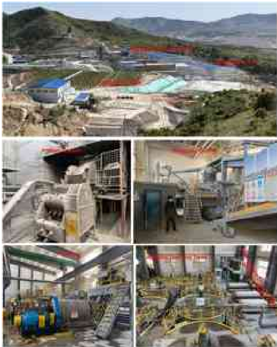
Figure 11-2: Site Photos of #1 Jilong Plant
